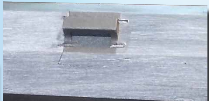
Barrel lug installed.
