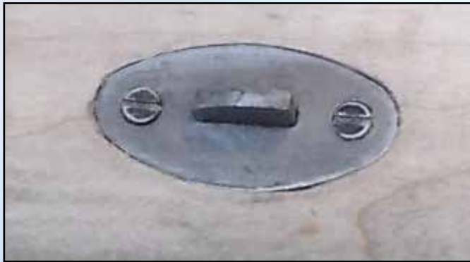
Barrel key escutcheon installed.
